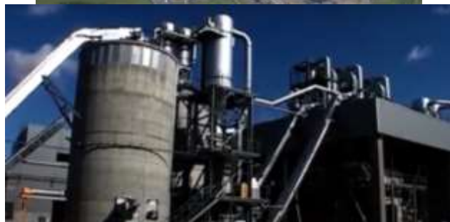
Biomass thermal power plant, Rădăuți city, Suceava County. General view
