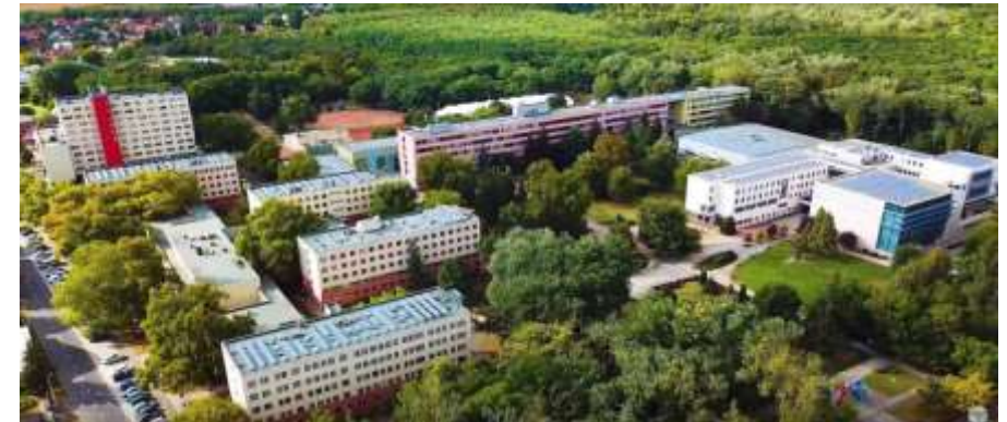
Aerial view of the campus, showing the PV panels installed on the roof of most buildings
