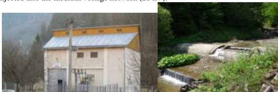
Micro-hydroelectric power plant on the river Barnar – general view of the main building
